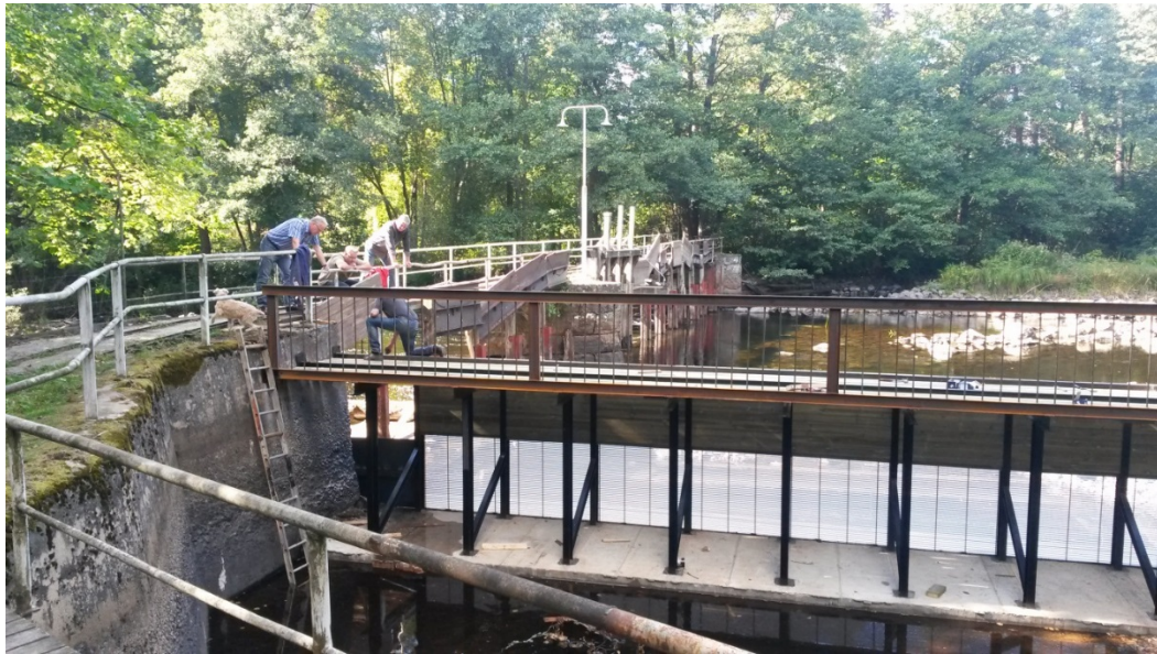
Figure 2. Construction of the smolt leader/diverter at Strömsbro. The steel rods prevent smolts from entering the inlet channel to the power plant. The photo is taken from the inlet channel. The dam construction with fishways for smolts and adults, a smolt trap and equipment for counting adults and registering PIT tags can be seen in the background.
