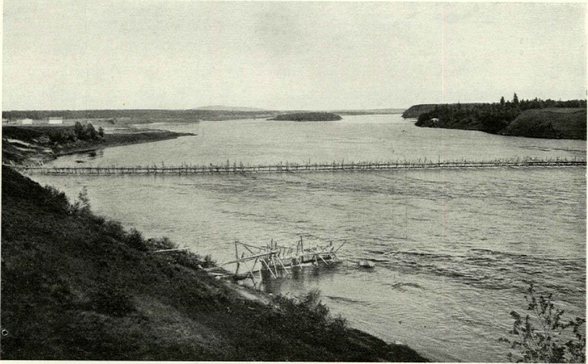
Fig. 14b. Kõngäs Fyke-Weir at the Point where the Kemi River branches. Small Bank Weir in Foreground.
